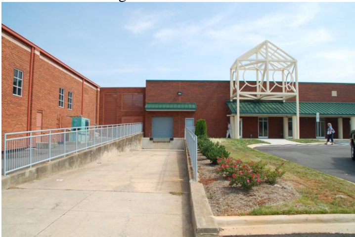
South Side Loading Dock:
